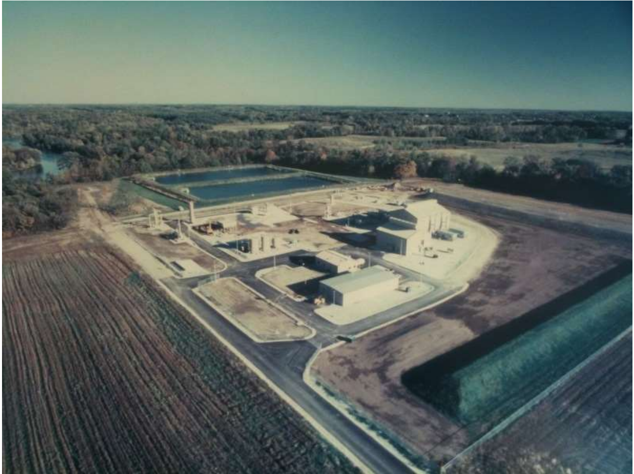
Eaton Rapids Gas Storage Facility; Eaton Rapids, MI; In-Service June 1989
