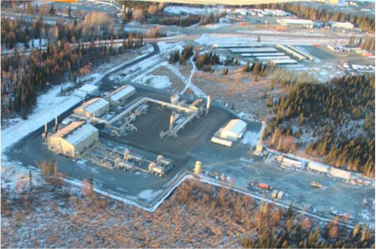
Cook Inlet Natural Gas Storage Facility; Kenai, Alaska; In-Service April 2012
